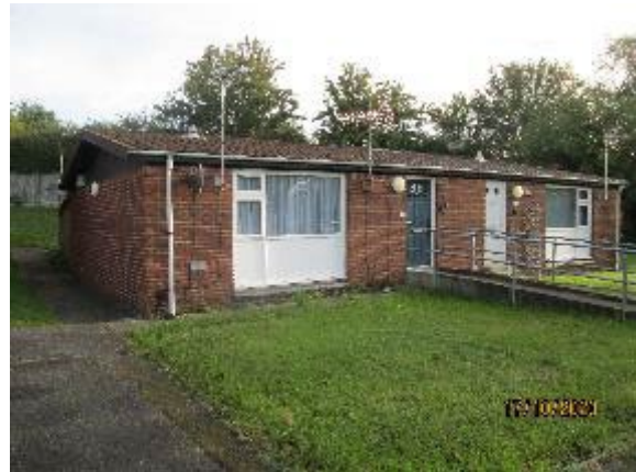
Principal elevation of the semi detached bungalow
