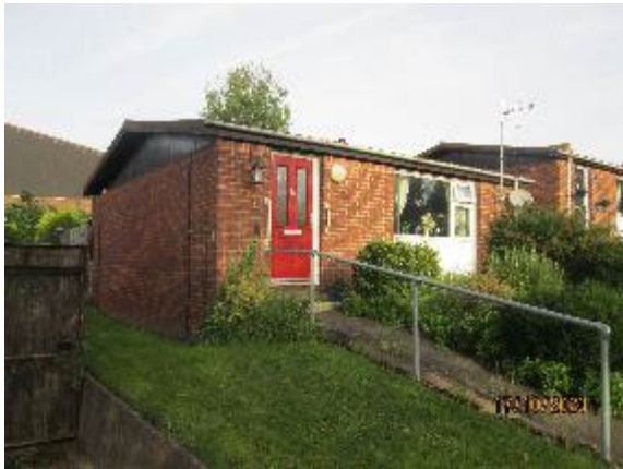
Principal elevation of the detached bungalow
